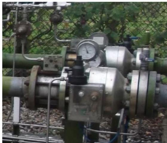
Two per stream, 100mm nominal size ‘IGA – Axial Flow’ regulators, configured for 2 stage pressure reduction.
