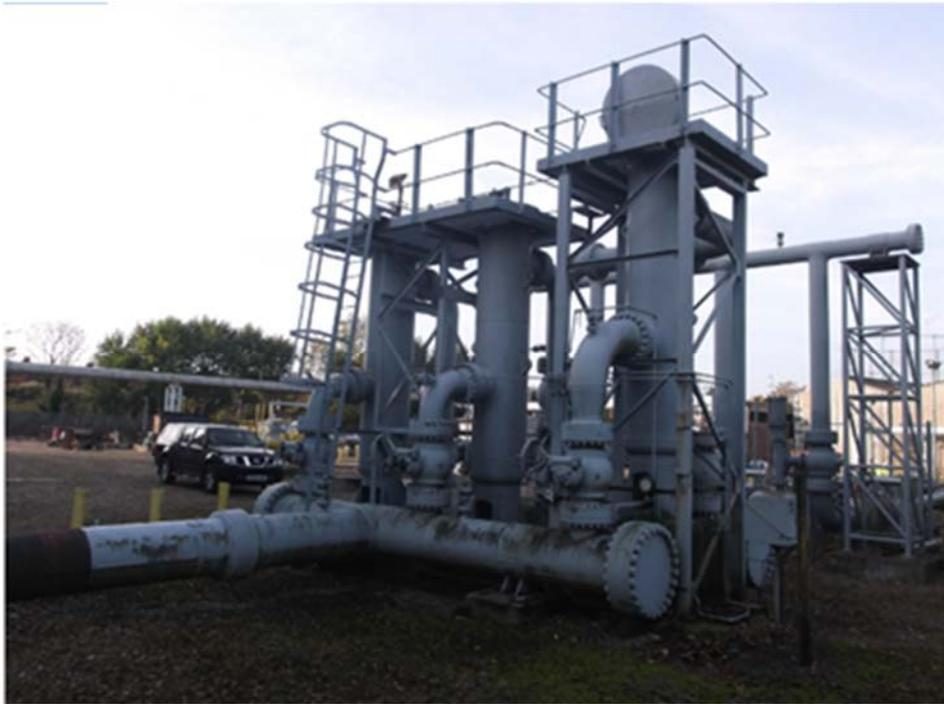
Figure 4: 'A' System vertical tower filters
