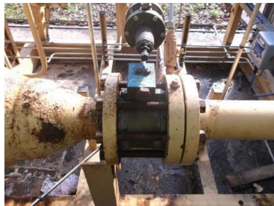
Second stage pressure reducing regulator
