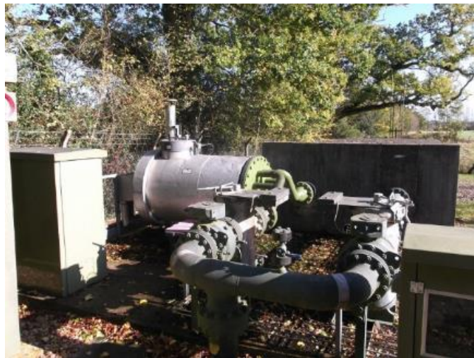
An elevation of the WBH with thermal insulation
