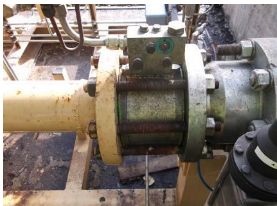
First stage pressure reducing regulator
