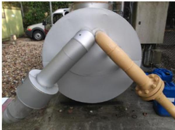
*38 BarG flow and return gas pipework*
