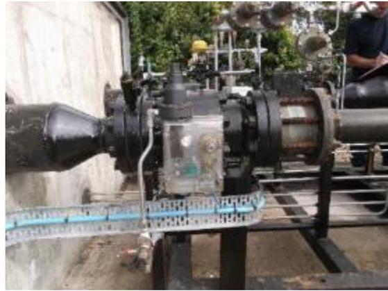
Two per stream, 100mm nominal size ‘IGA – Axial Flow’ regulators, configured for 2 stage pressure reduction.
