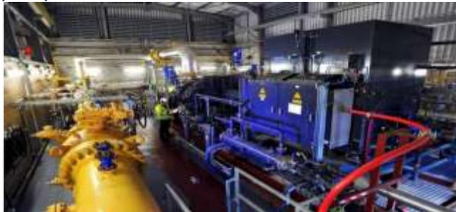
The system has been in operation for the past five years and will have run some 40,000 hours and is reaching its half-life point. The system onsite consists of dual redundancy 24v battery charger units feeding the low voltage control and SIL2 rated protection loops with a 230v UPS system feeding the site PC, the emergency shutdown shut system and human machine interface, providing fault data logging and a system overview.
