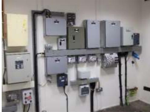
A number of SGN's electrical kit contains asbestos as this material was used within fused switchgear, fuse boards or behind ceramic fuses. A lot of SGN's older electrical kit does not allow equipment to be safely isolated using SGN Safe Isolation Procedure.
